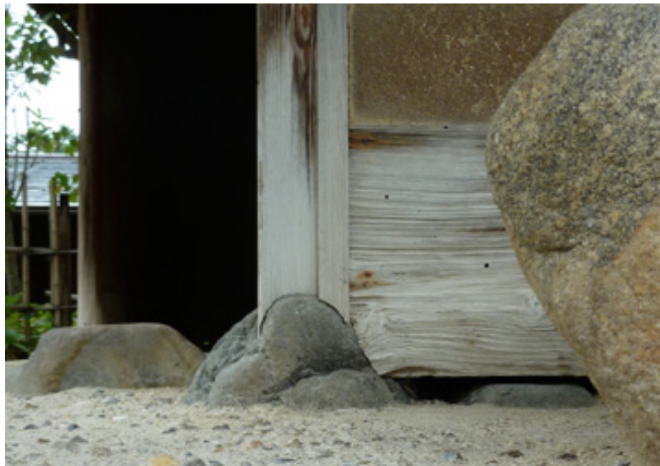
Fig.28. Wall/Floor architectural detail on a traditional Japanese teahouse 1 Photograph by James Kirk The unsuitability of this rounded stone as a foundation for the small building would be considered problematic in the West.
